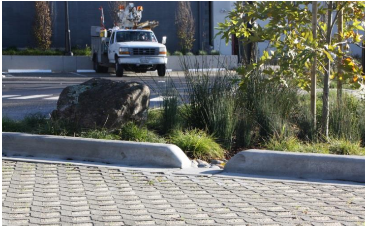
Parking lot with permeable paving and rain gardens
