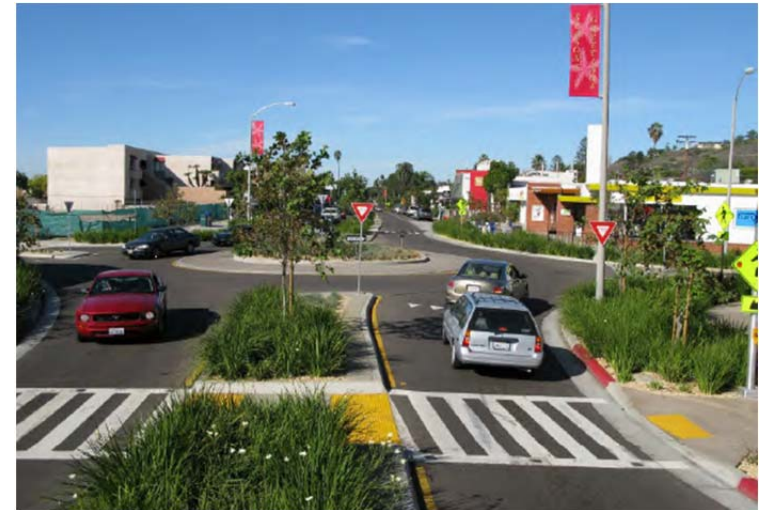
Pedestrian refuge islands provide a protected resting place for pedestrians when crossing wider streets – approximately more than two lanes of traffic
