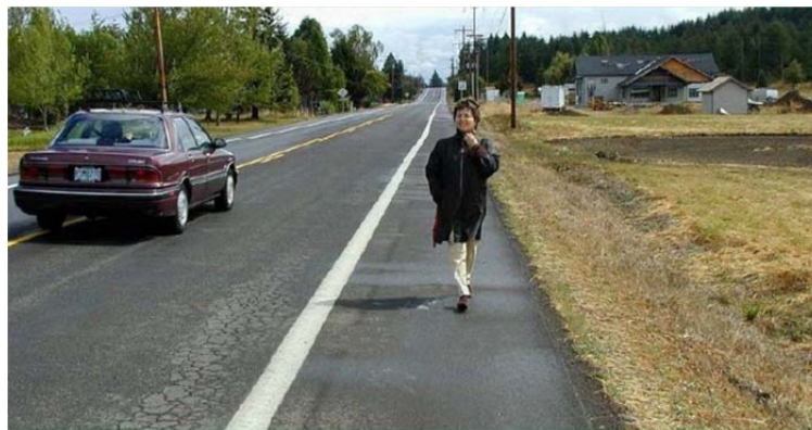
Paved shoulders (6 feet preferred) provide safe walking areas for pedestrians along Rural Connectors and can also improve safety for cyclists
