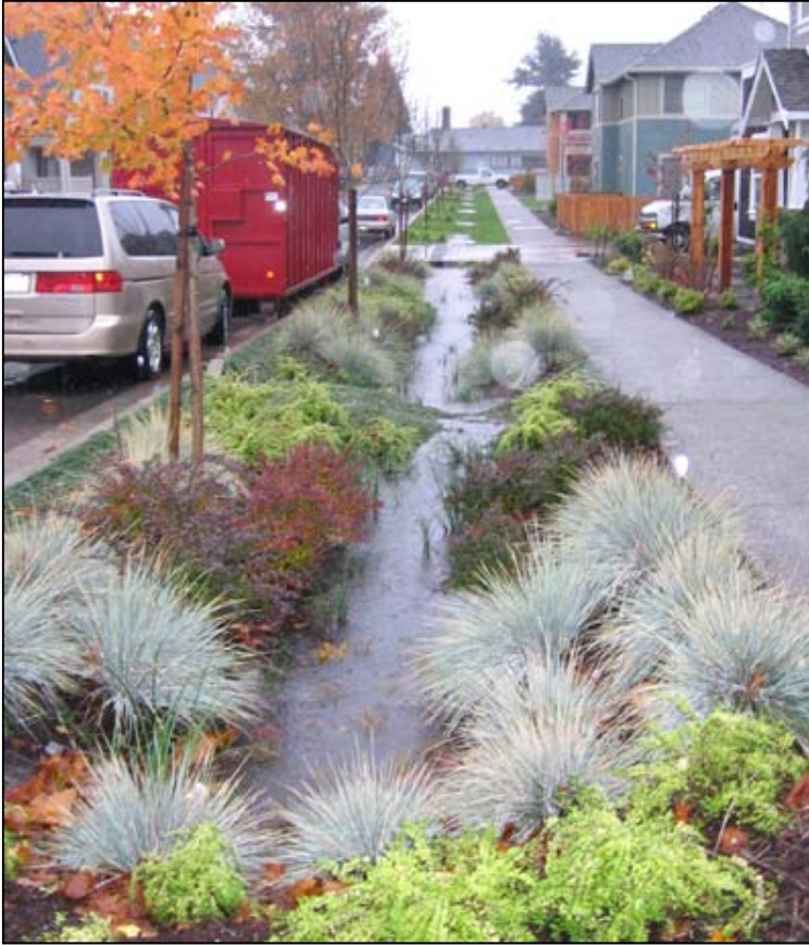
A bioswale is a wide depressed channel that collects and infiltrates stormwater rather than directing it to a drainpipe, reducing run-off and improving water quality.
